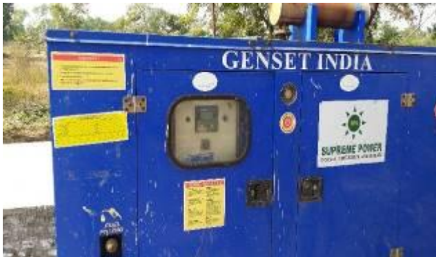
Gen set at WTP. In case of non Green DG testing of emission is required
