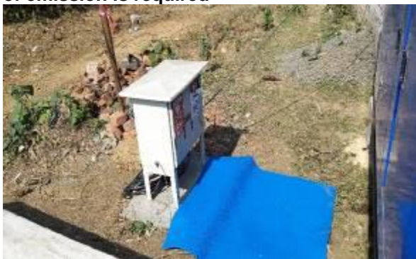
Rubber mat noted below main switch board
